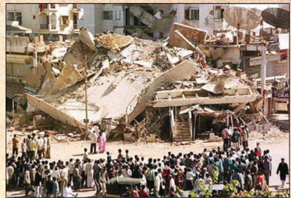
Fig. 3.7 : Destruction caused by Bhuj Earthquake
